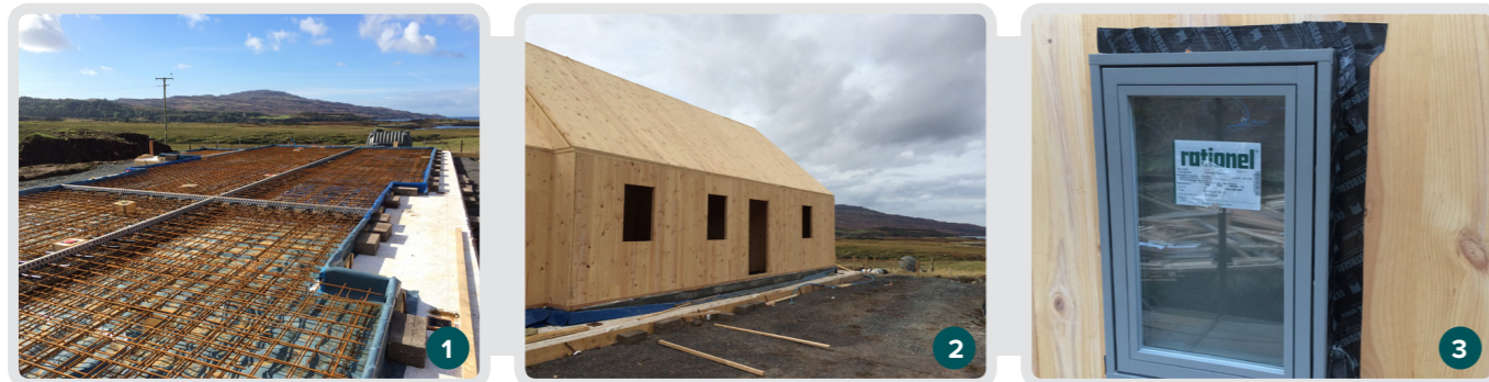
1 Wire mesh in place to reinforce the concrete structural slab, below this is a DPM and 250mm Filcor 45 under-slab insulation; 2 the houses were built with cross laminated timber panels which provide strength, reduced construction time, and can help in minimising thermal bridges; 3 windows are Rationel triple glazed units with Extoseal Encors tape for sealing to the CLT panels
